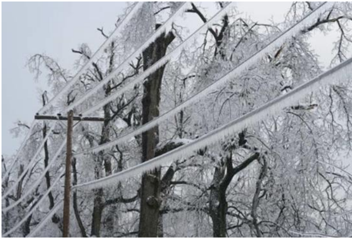
Figure 26: Ice Covered Power Lines
